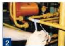
2 remove paint and clean pipe
