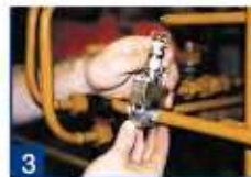
3 clamp SC onto pipe
