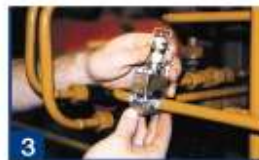
clamp SC onto pipe
