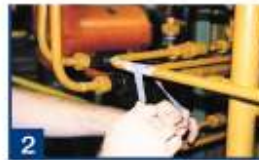
remove paint and clean pipe
