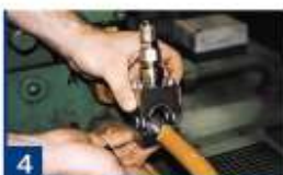
clamp SC onto pipe
